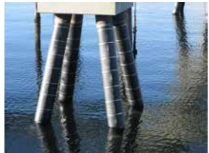
Repair and protection for a pump housing with epoxy filled with ceramics.
