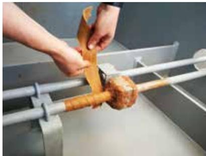
**TidalWrap anti-corrosion tape for pillars.**
