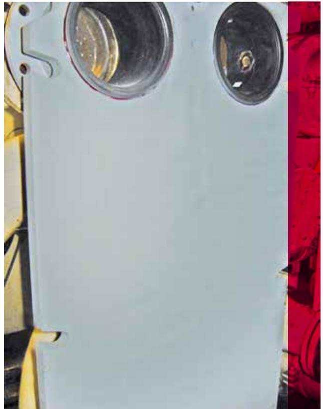
**Repair to the cover of a heat exchanger with Devcon Titanium.**
